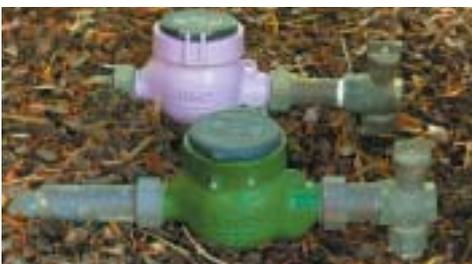
Recycled water is supplied to your home in a separate pipe. Recycled water is supplied through the lilac coloured meter at your property boundary. The drinking water meter is coloured green. From the lilac meter water is distributed through the lilac coloured pipe system.
