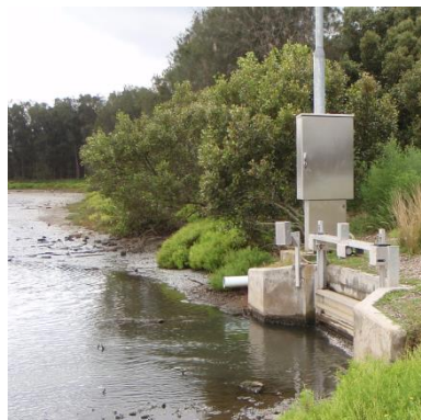
Tidal flushing has been restored to landlocked estuarine wetlands. Inundation is managed seasonally to control algal growth and to balance migratory shorebird, saltmarsh, mangrove and mosquito needs
