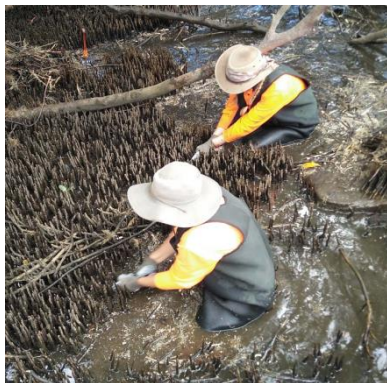
Mangrove drainage channels are hand-cleared to maintain tidal flows and thus prevent ponding and dieback
