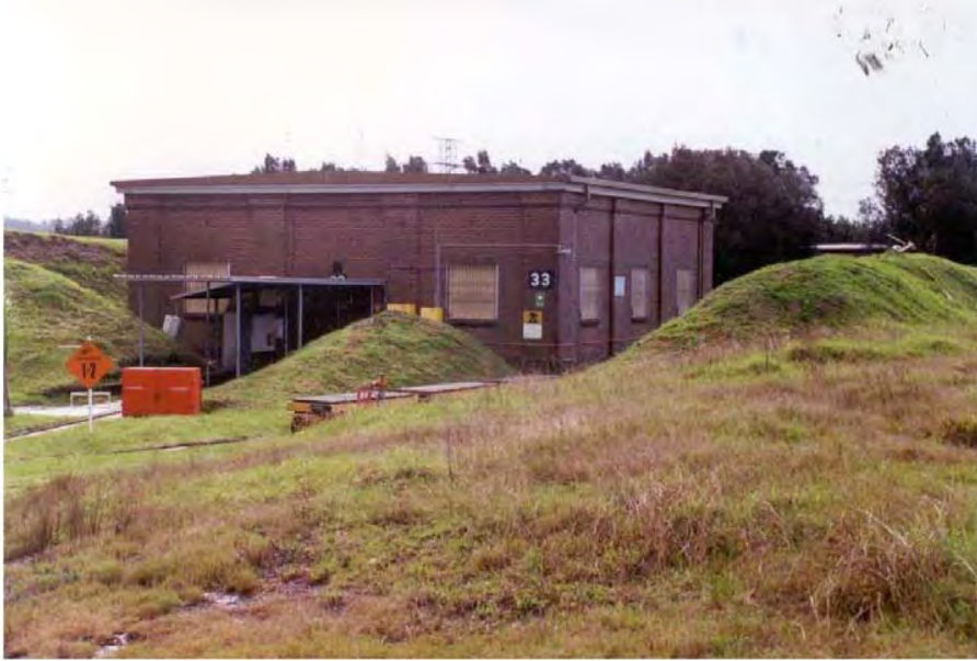
Figure 3-32 RAN pre-WWII explosives storehouse (33).
