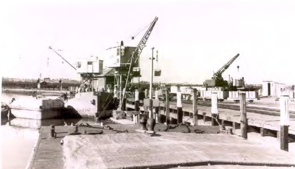
Figure 3-24 Cranes, lighters and rail transport on the wharf, 1950s (Schwager Brooks and Partners 1996).
