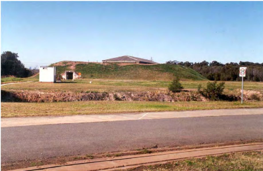
Figure 3-33 Large RAN Explosives Storehouse (18) protected by earth traverse (Schwager Brooks and Partners).
