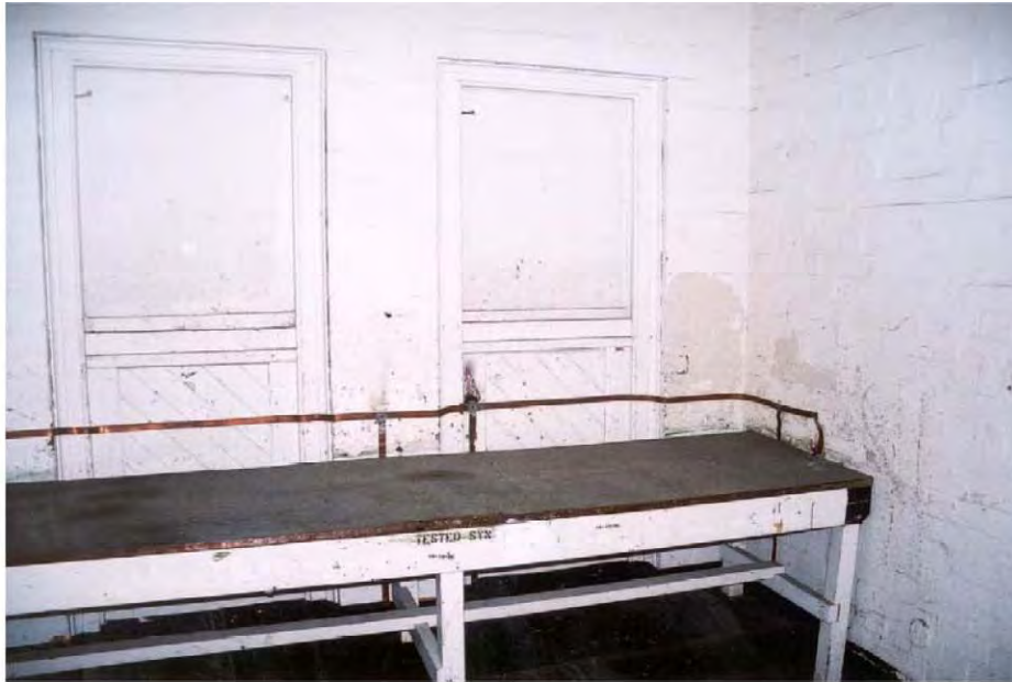
Figure 3-27 Benches and equipment in workshops are securely earthed (Schwager Brooks and Partners 1996).
