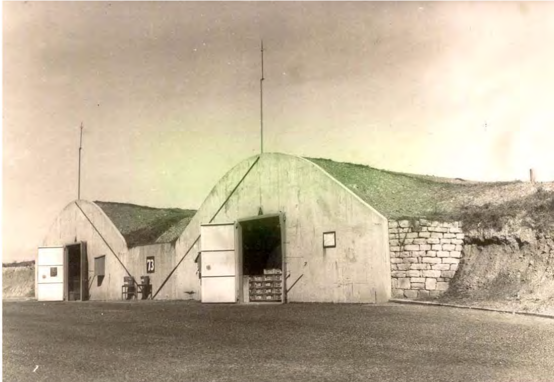
Figure 3-34 US Navy storehouses under earth berms. The buildings (No. 73) have been demolished. (Schwager Brooks and Partners, 1996).
