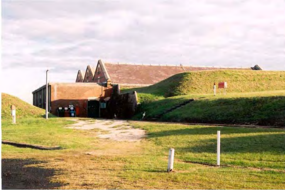
Figure 3-5 Original Gun Powder Magazine (20) with protective earthworks.
