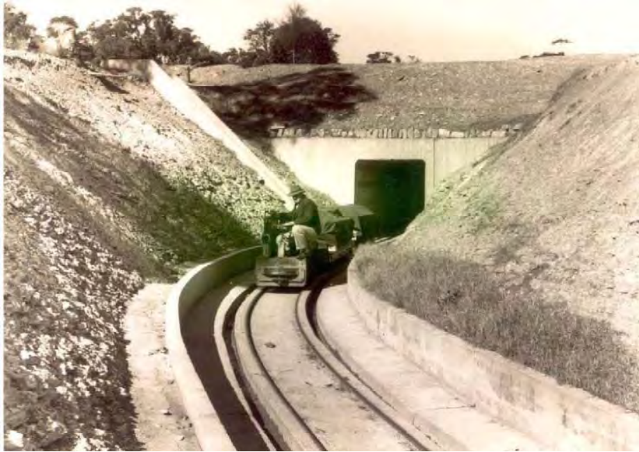
Figure 3-22 Electromobile and trolleys in cutting, 1950s (Schwager Brooks and Partners 1996).
