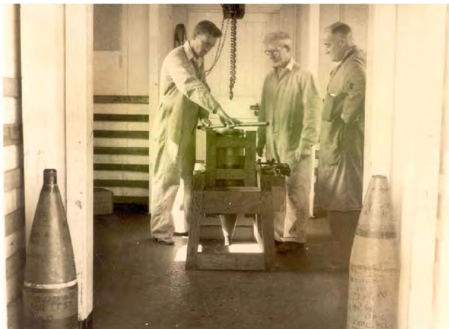
Figure 3-19 Examination of a Shell Fuse, 1950s (Schwager Brooks and Partners, 1996).
