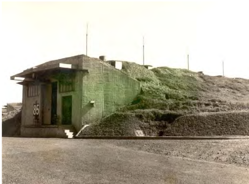
Figure 3-35 Former single concrete box style underground explosives storehouse (85) now demolished (Schwager Brooks and Partners 1996).
