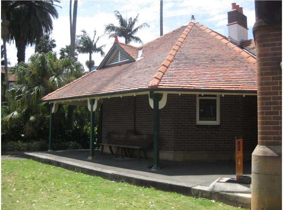
Figure 99 North verandah, Gatehouse, Building E
