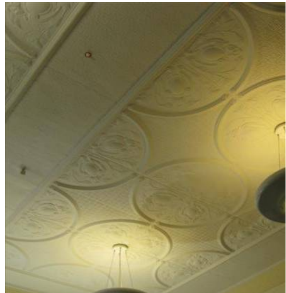
Figure 60 Detail, pressed metal ceiling, ground floor
