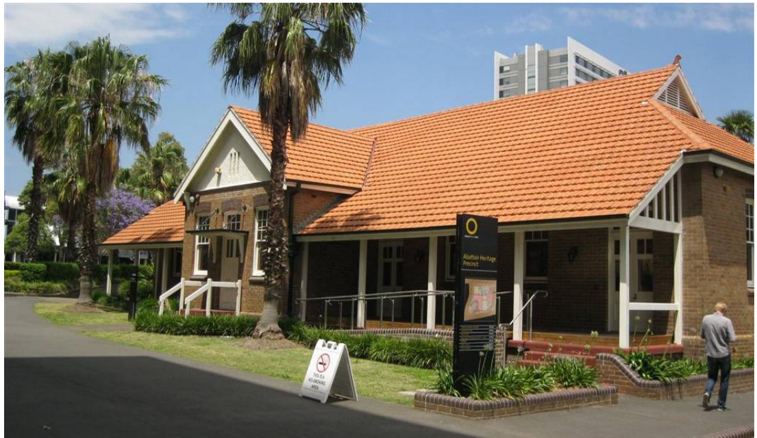
Figure 70 Eastern elevation of Building B
