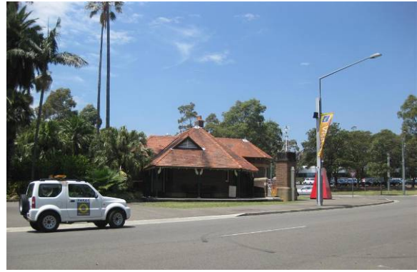
Figure 20 View to Building E from Showground Road
