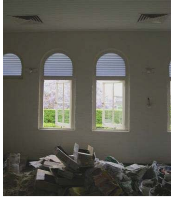
Figure 86 Interior during construction
