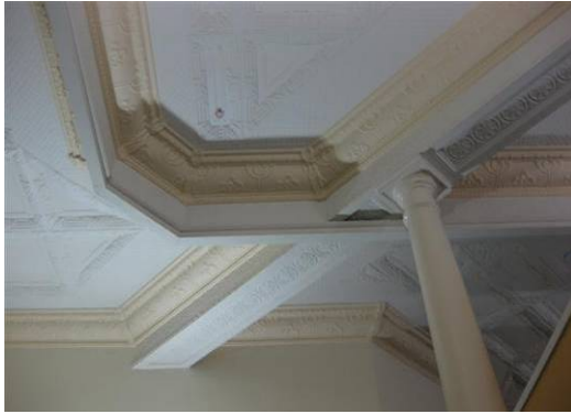
Figure 61 Pressed metal ceiling, lobby
