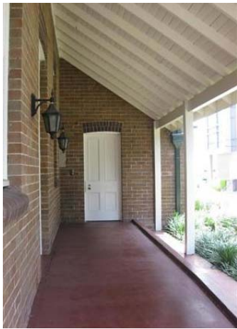
Figure 73 South eastern verandah
