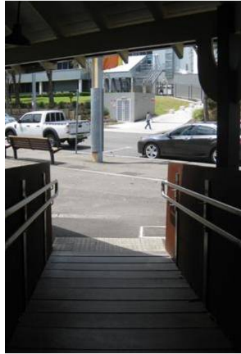
Figure 103 Access ramp, looking out
