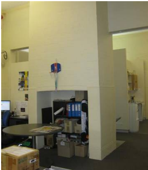
Figure 59 Former fireplace, ground floor
