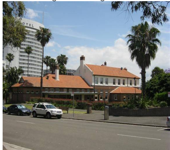
Figure 22 View to Building A from Herb Elliott Avenue
