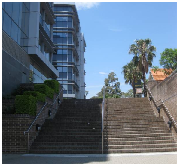
Figure 11 View south along eastern boundary of the site. Commonwealth Bank Building is on the left.
