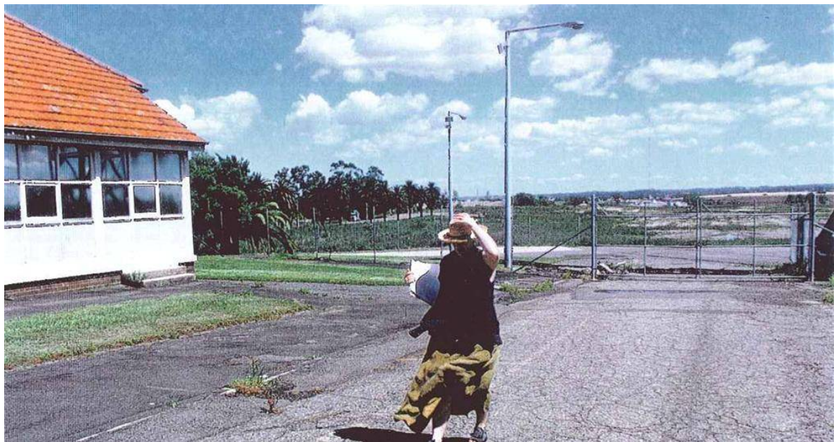
Figure 146 Eastern façade of Building B. 1995 Source: Conservation Study, Playfair Memorial Fountain Homebush, 1995
