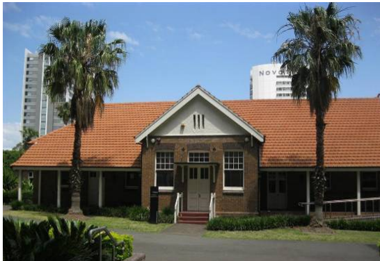
Figure 44 Garden beds in front of Building B
