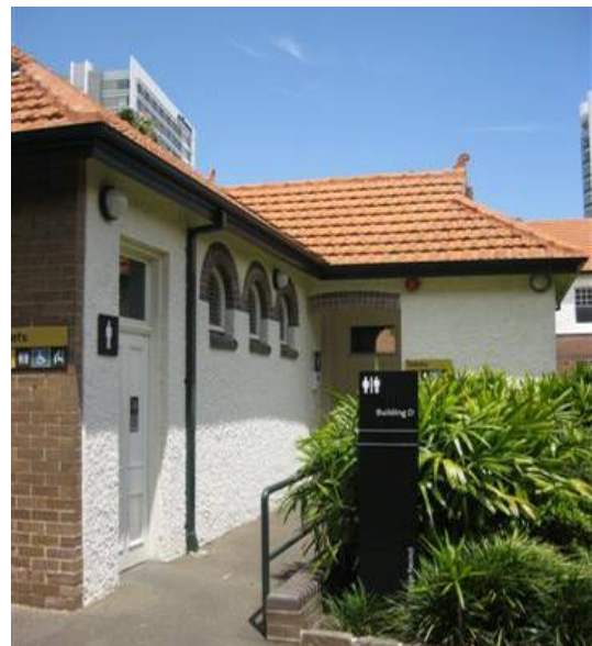
Figure 92 Northern wall, with ramp to accessible and ladies toilets
