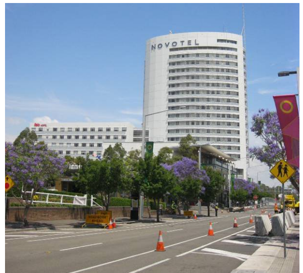
Figure 12 View west along the northern boundary of the site, showing the retaining wall along the edge of Dawn Fraser Avenue and looking towards the Hotel Ibis & the Novotel
