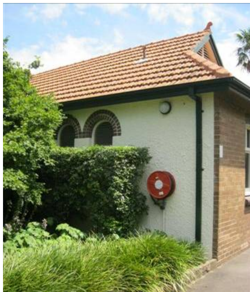
Figure 91 Southern wall, showing detail of roughcast render and brick arched openings
