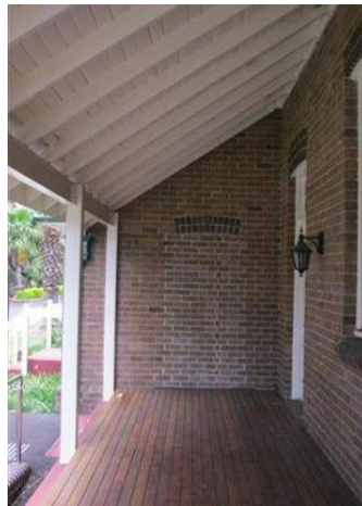
Figure 74 North eastern verandah
