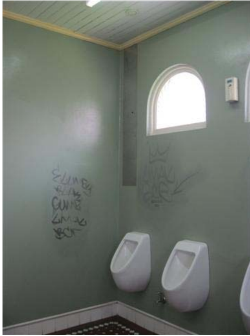
Figure 93 Interior, Mens Toilets
