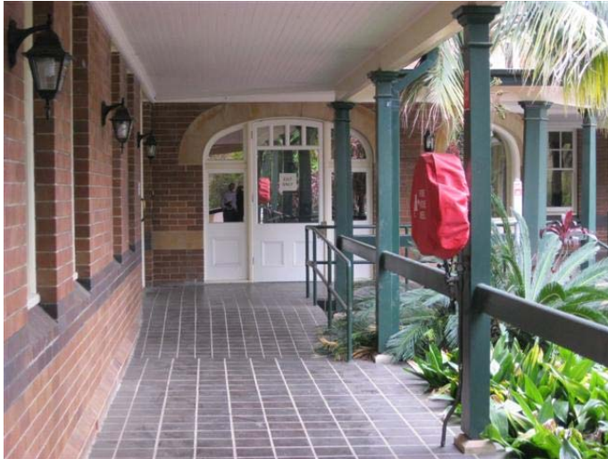
Figure 56 Front verandah. Note level changes to provide equitable access.
