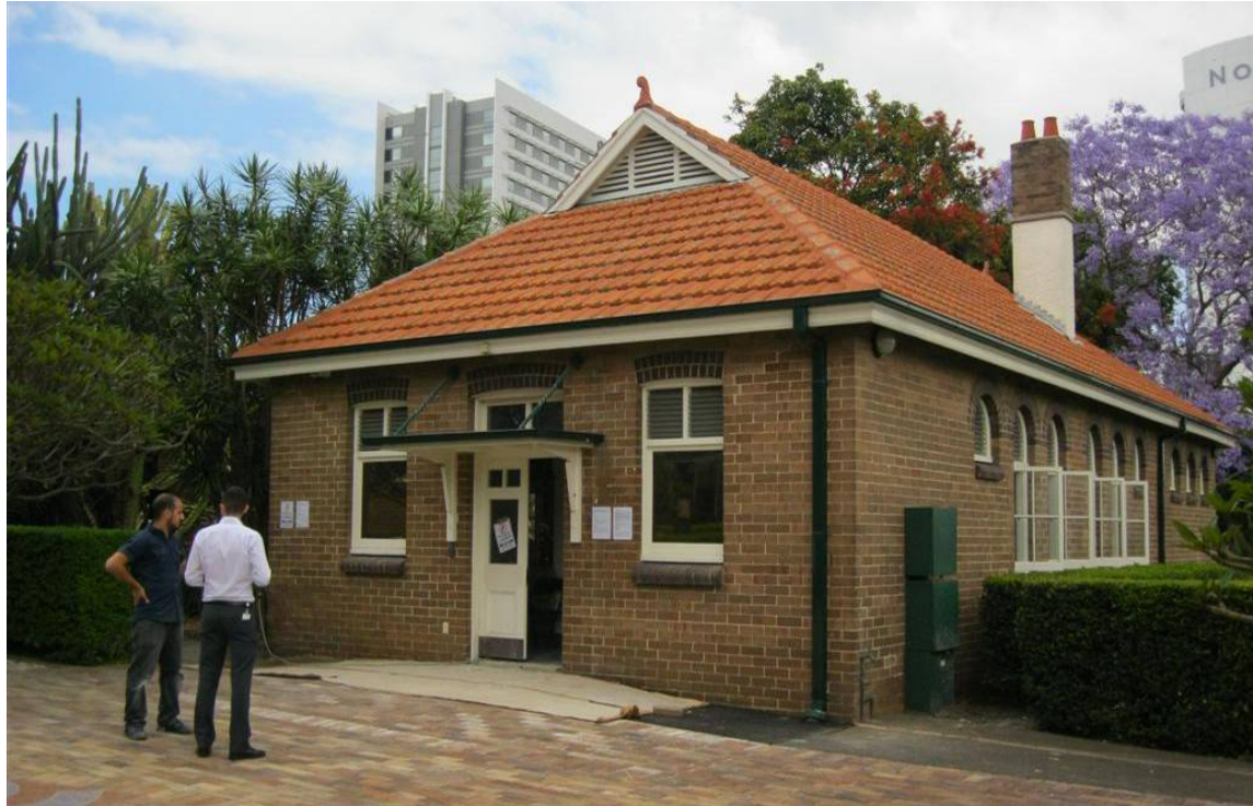
Figure 82 Eastern façade of Building C
