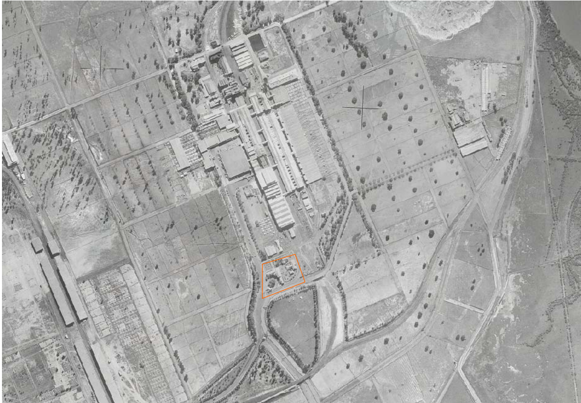
Figure 133 Aerial view of the State Abattoirs, 1943 Source: Six Viewer
