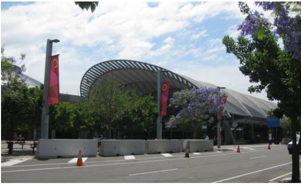
Figure 15 View to Railway Station, north of the site
