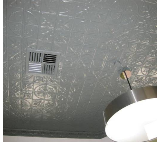
Figure 108 Pressed metal ceiling
