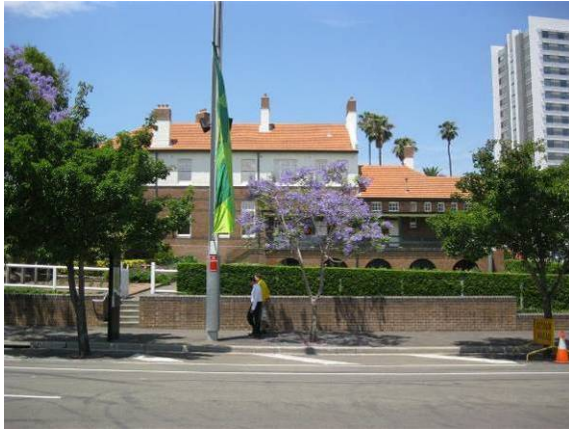
Figure 23 View to Building A from Dawn Fraser Avenue. Note the retaining wall.
