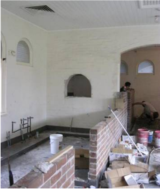
Figure 85 Interior, during construction of café
