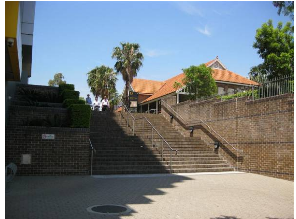
Figure 24 View to Building B along eastern boundary. Note the retaining wall along the northern edge of the precinct.
