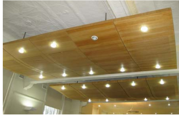
Figure 62 Modern timber ceiling, ground floor board room
