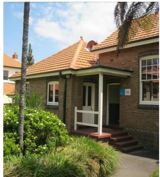
Figure 72 Rear porch, Building B
