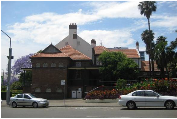
Figure 19 View to Building A from Showground Road
