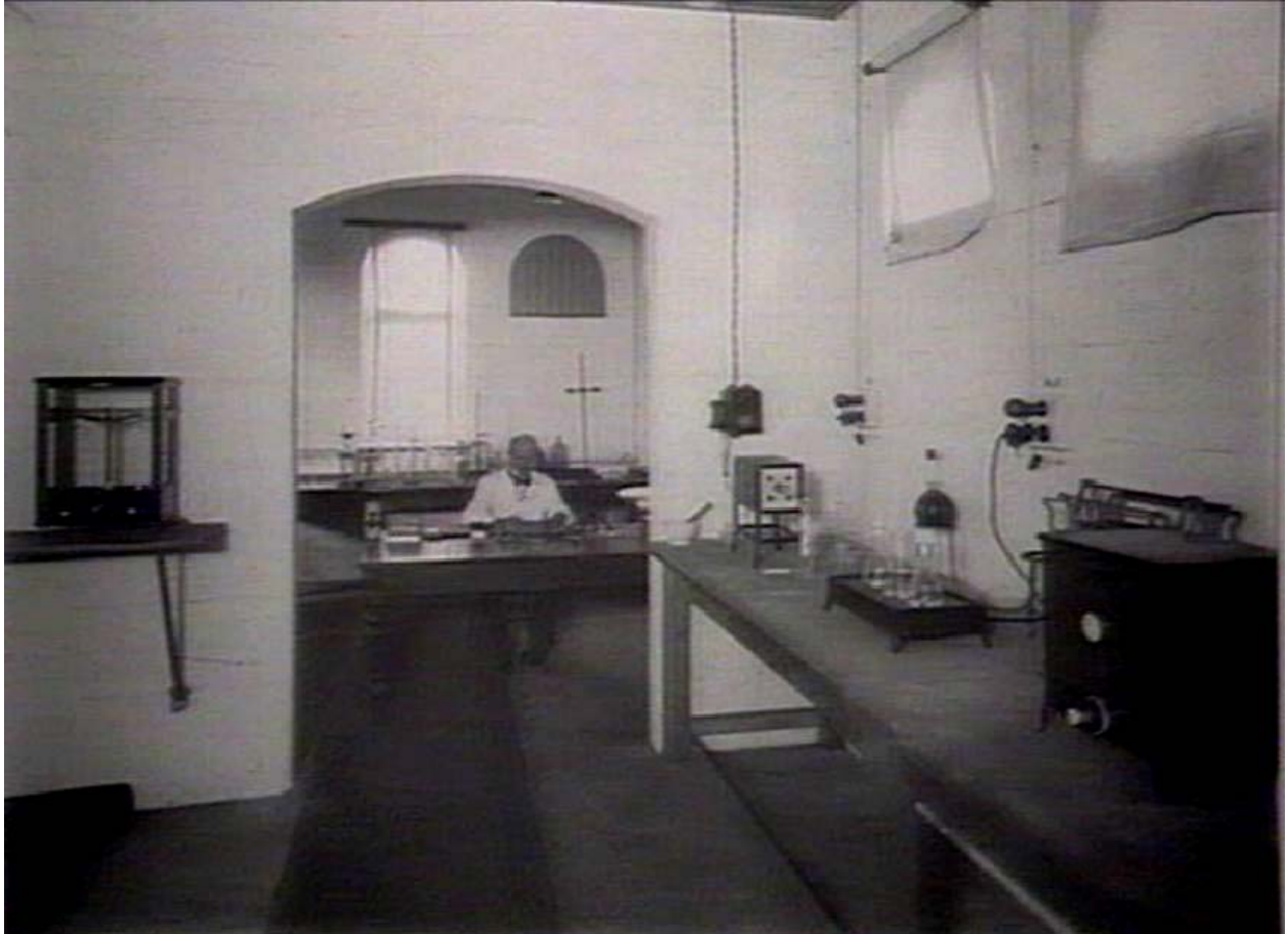
Figure 131 1947 photograph showing inside the laboratory building Source: State Library of NSW
