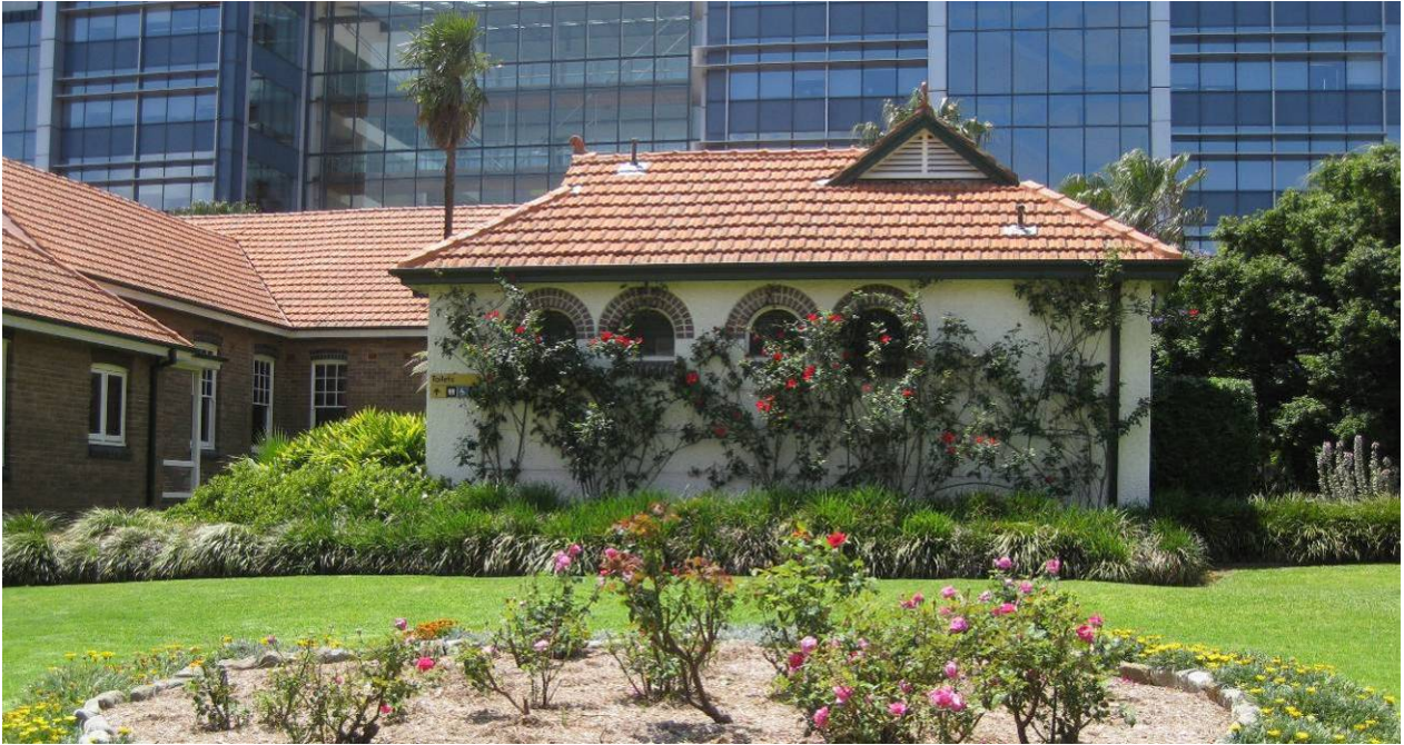
Figure 90 Western elevation of Building D, showing roughcast render and high-level brick-edged windows
