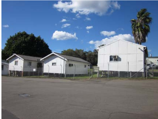
Figure 3-72 Buildings 2, 3 and 197, situated close to the Jamieson Street entry to the site (Source: Tanner Architects).
