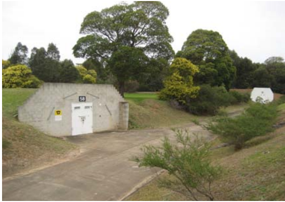
Figure 3-25 The construction of explosives stores and associated road access generated the industrial landscape associated with the Armory in the southern part of the US Navy Utilisation Precinct (Source: Tanner Architects).
