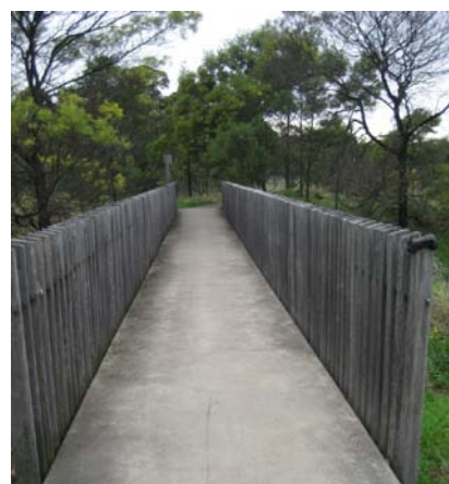
Figure 3-68 A recently constructed bridge at the southern end of the precinct (Source: Tanner Architects).
