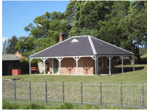
Figure 3-41 Building 139. Intrusive verandah infills evident in 1996 photographs have since been removed and the verandahs reconstructed (Source: Tanner Architects).
