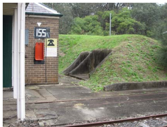
Figure 3-56 Bunkers cut into the berm on the south side of Building 155. The signage on the wall of the building is characteristic and is important in understanding the operations of the Armory (Source: Tanner Architects).
