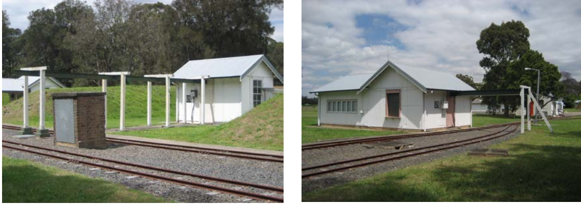
Figure 3-50 Buildings 128 (left) and 129 (right) are components of a small group of buildings originally used for inspection and testing, and demonstrate the close links between buildings and infrastructure, in this case the light rail, that are one of the important characteristics of the Armament Depot (Source: Tanner Architects).
