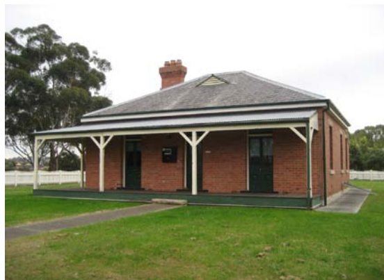
Figure 3-39 Former residence, Building 123. The verandah has been reconstructed – photographs taken in 1996 show it had been removed before that time. The building is now part of Sydney Olympic Park Lodge (Source: Tanner Architects).
