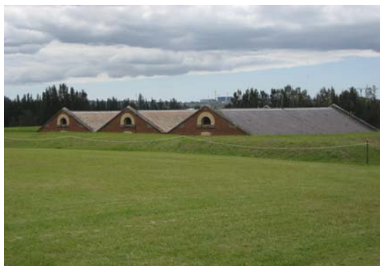
Figure 3-36 Building 20 viewed from the west graphically demonstrates the procedure of containing explosions through earthworks. The roof form of this building is the most distinctive built element on the site (Source: Tanner Architects).
