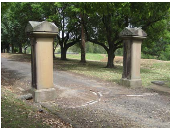
Figure 3-34 Late nineteenth century stone gateposts, with the early road beyond (Source: Tanner Architects).
