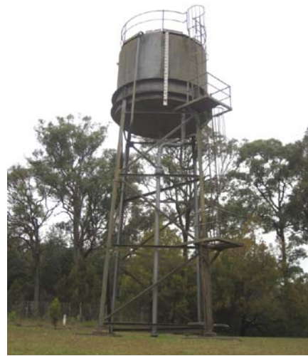
Figure 3-52 Water tower Building 196 (Source: Tanner Architects).
