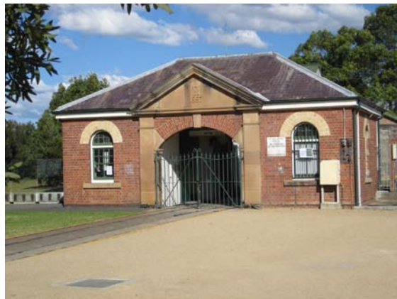
Figure 3-33 Building 143, the gatehouse, is amongst the most architecturally considered buildings within the site (Source: Tanner Architects).
