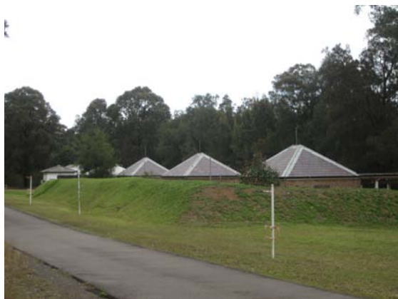
Figure 3-53 The roofs of Buildings 55, 56 and 57 rise above the protective berm (Source: Tanner Architects).
