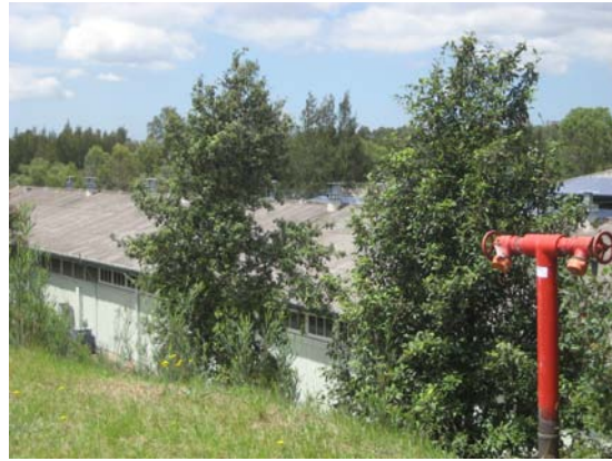
Figure 3-66 Building 46 viewed from the top of the surrounding berm (Source: Tanner Architects).
