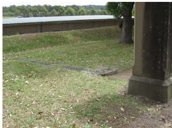
Figure 3-35 Footings of early fence. Other footings extend across open ground to the east of the gateposts (Source: Tanner Architects).
