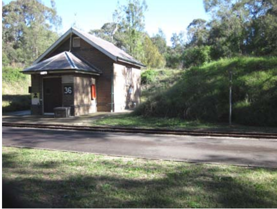
Figure 3-57 Buildings 36, 37 and 38 are similar in appearance although Building 38 is larger than the other two (Source: Tanner Architects).
