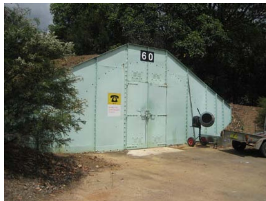
Figure 3-71 Several of the storehouses feature steel “facades” (Source: Tanner Architects).
