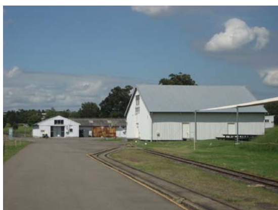
Figure 3-46 Building 22 (the Armory Theatre), which occupies an important location at Five Ways. Building 24 is visible beyond it (Source: Tanner Architects).
