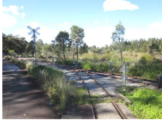
Figure 3-63 Light rail tracks at the southern end of the precinct (Source: Tanner Architects).
