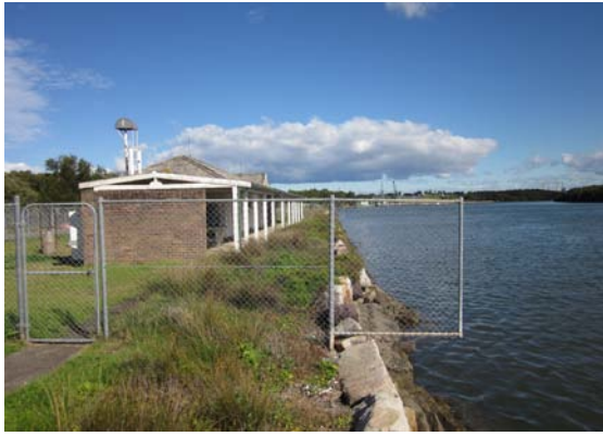
Figure 3-48 Reclaimed foreshore and Building 193 (Source: Tanner Architects).
