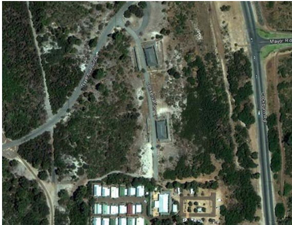
Figure 4-12 Woodman Point retains three large magazine buildings, with one reused as the caravan park administration building at the lower end of the photograph (Source: Google Earth).
