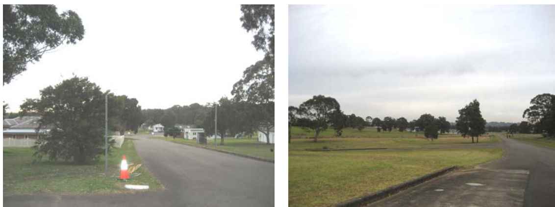
Figure 3-29 Roads, as well as being significant infrastructure, are also important defining and unifying elements within the site. The road extending east from the Jamieson Street entry, at left, defines the Original Establishment and US Navy Utilisation Precincts, while the Burma Road, at right, links all four precincts and is the major pathway through the site (Source: Tanner Architects).
