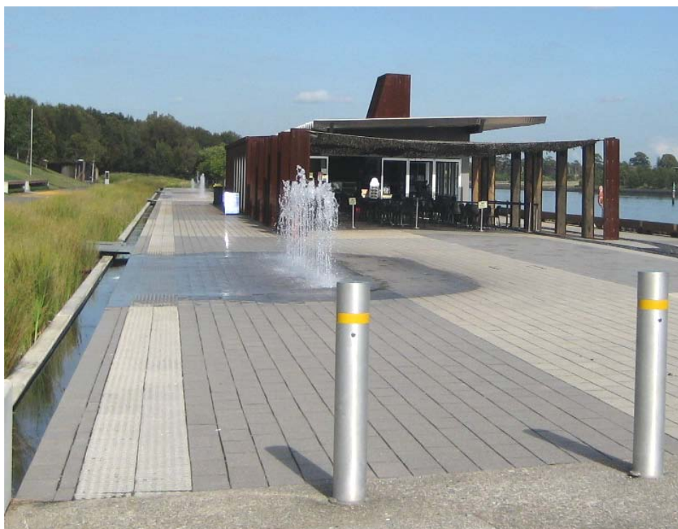
Figure 2-11 Rebuilt Armory Café, 2009 (Source: Tanner Architects).
