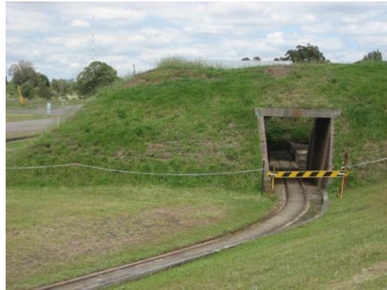
Figure 3-43 Building 20 is totally enclosed by a high berm, with light rail access cutting through it (Source: Tanner Architects).
