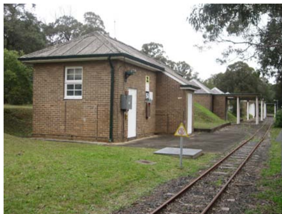
Figure 3-54 Former soldering room, Building 154, with the group of workshops Buildings 155-157 beyond (Source: Tanner Architects).
